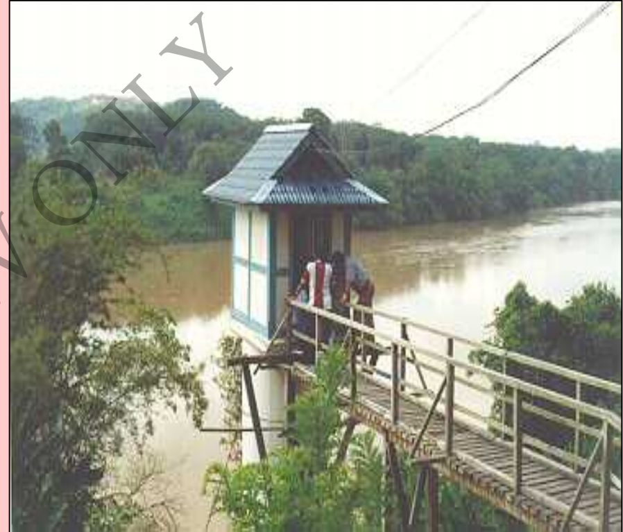
RIVER LEVEL TELEMETRY STATION ( 224 pcs )
